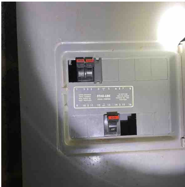
9.6.6 The HVAC service disconnect was located within line of sight of the unit as required. (Exterior Back)
